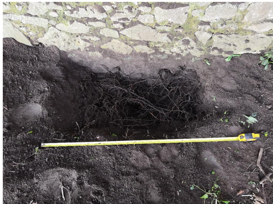
Fibrous roots contained in the upper 200-400mm of soil, that have grown through cracks in the stone wall.
