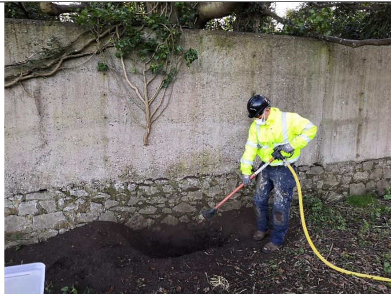
Excavations at the base of boundary stone wall.
